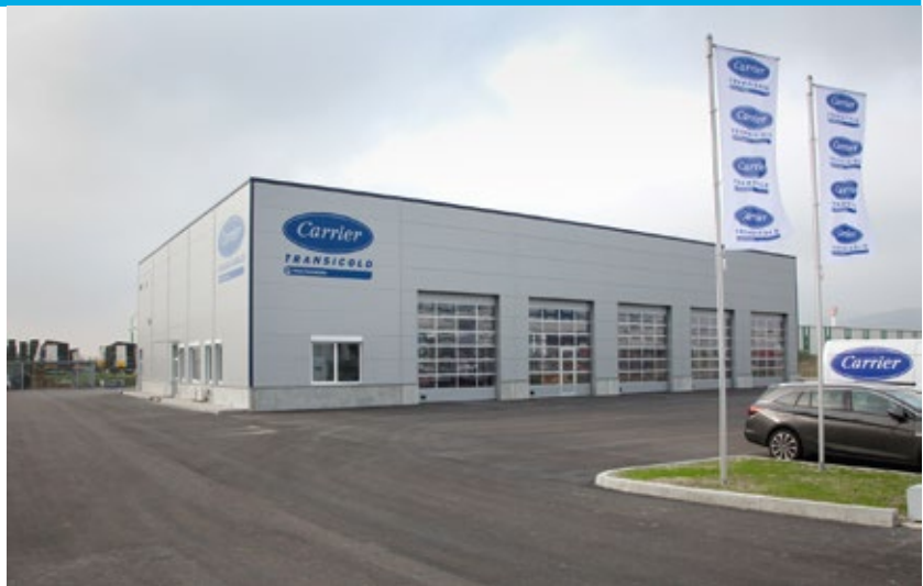
Die neue Carrier Servicestation in Wiener Neudorf.
